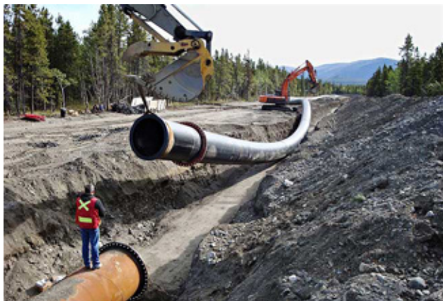
Atlin Hydro penstock installation, Taku River Tlingit First Nation, BC
