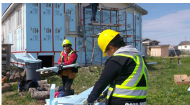
Local workforce adding insulations and air sealing a home on the James Bay coast. Photo Credit: Conservation on the Coast Facebook.
