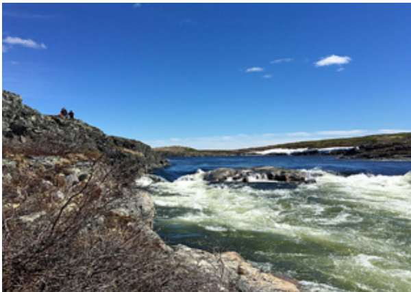
The future site of the 10MW Innalik Hydro project on the Inukjuak River.
