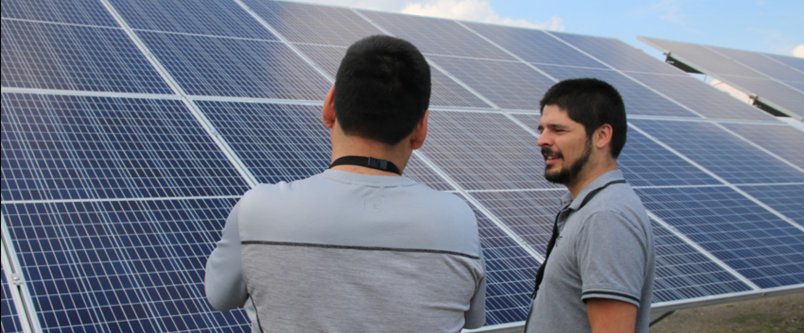
2019 Catalysts Tour of Nanticoke Solar built on the recommissioned site of one of Canada's largest coal plants with partnership with Six Nations of the Grand River and the Mississaugas of the Credit First Nation.
