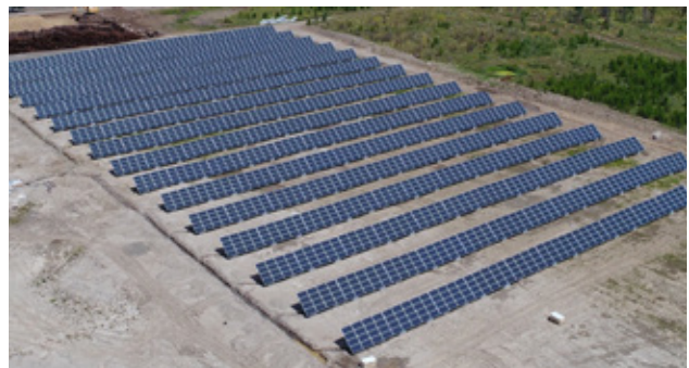
An aerial view of the Tsilhqot'in First Nation's solar array. Photo credit: EcoSmart.
