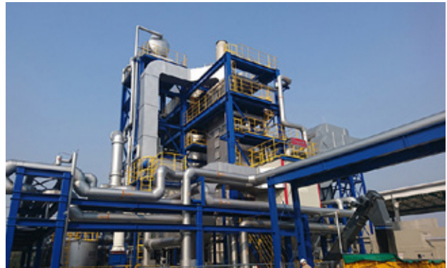
Meadow Lake Tribal Council set to construct an Organic Rankin Cycle facility like the one pictured here. Photo credit: Meadow Lake Tribal Council Bioenergy Centre.
