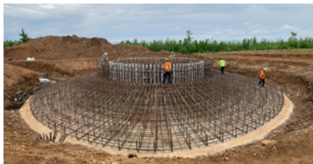
Workers building a platform for one of a dozen wind turbines as part of the Wocawson Wind project. Photo credit: Natural Forces.
