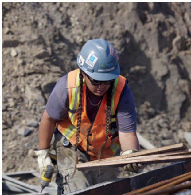
Mi'gmaq carpenter in the base of a wind turbine at the Mesgi'g Ugu's'n Wind Farm Photo: www.muwindfarm.com
