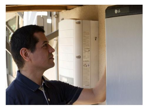
The system installed and tested by Pecan Street included seven (7) two-hour, 5kW batteries affixed to the outside of homes within Pecan Street's volunteer research network in Austin, TX.
