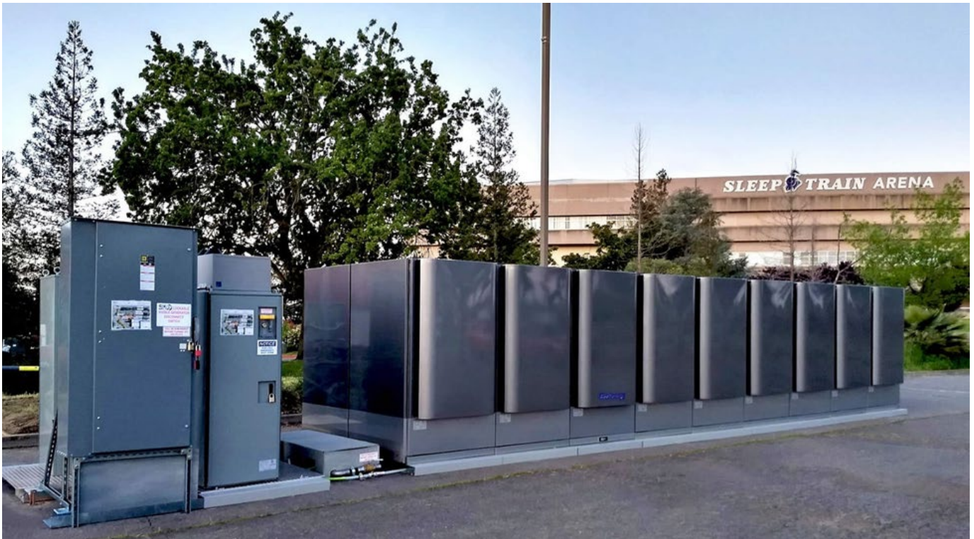
Figure 1: Bloom Microgrid powering temporary hospital at Sleep Train Arena in Sacramento
