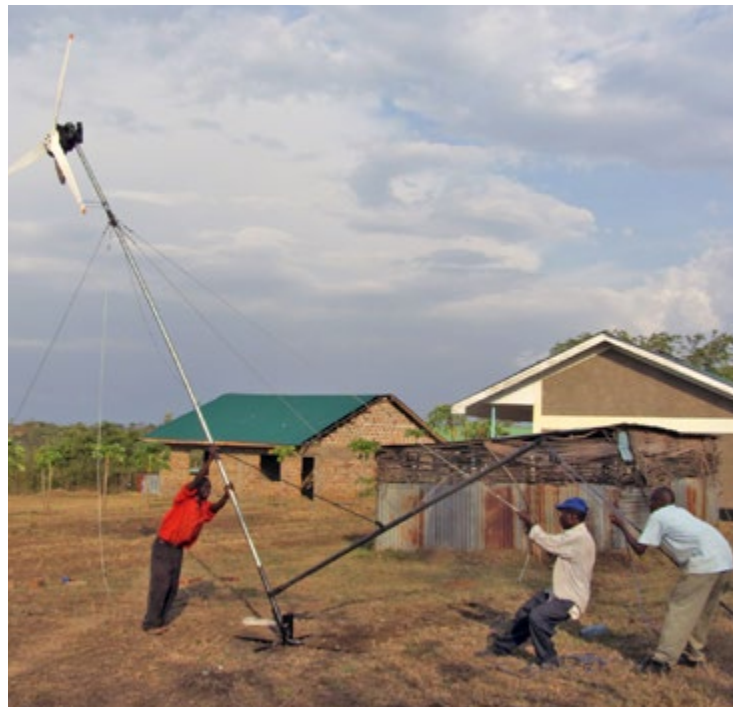
Installing a home-made wind turbine at a clinic in Homa Bay county.
