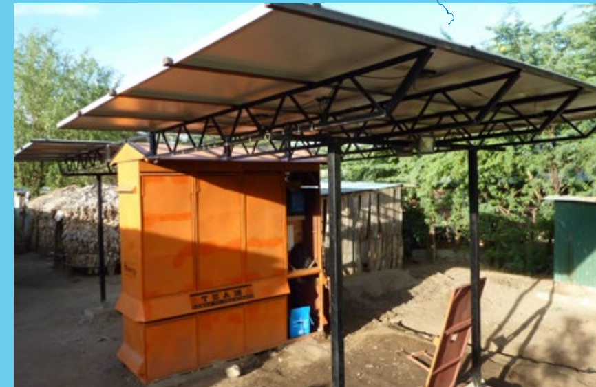
The Power Hub at Entesopia contains all the energy storage and control technology.
