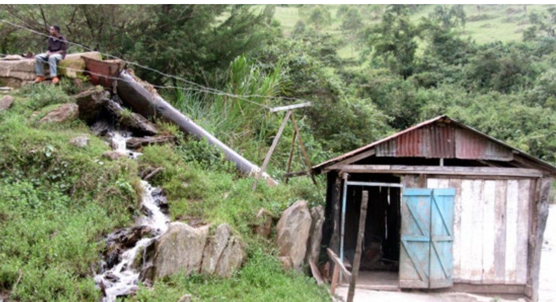
This home-made hydro-electric microgrid provides power to several houses, shops and a school.
